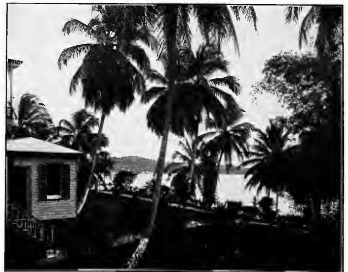
SANITARY OFFICE, BOCAS DEL TORO
